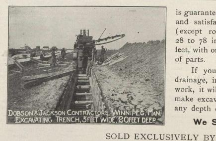
is guaranteed to work most economically and satisfactorily in any kind of soil (except rock), cutting any width from 28 to 78 inches and any depth to 20 feet, with one set of buckets, no change of parts.
