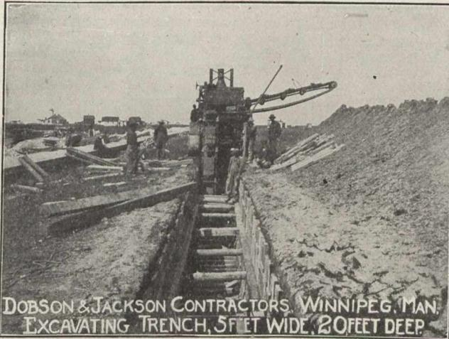
is guaranteed to work most economically and satisfactorily in any kind of soil (except rock), cutting any width from 28 to 78 inches and any depth to 20 feet, with one set of buckets, no change of parts.
