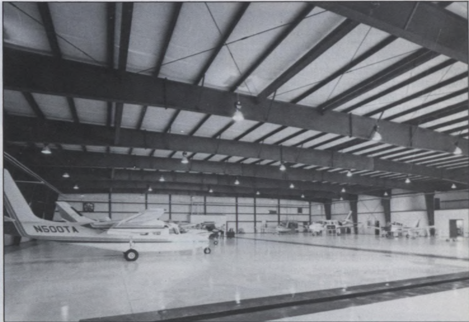
Pre-engineered aircraft hangar
