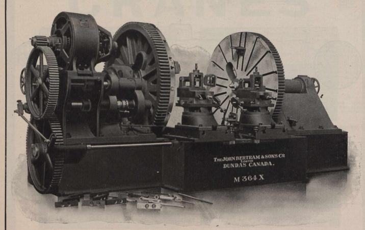
The illustration represents our new design Double Driving Wheel Lathe supplied the Intercolonial Railway. This lathe has an actual swing of 104 inches and is equipped with Patent Tool Holder and Teas Patent Drivers. Manufactured in sizes 80, 90 and 100-inch swing.
