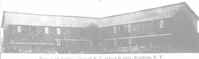
Amatite on Lumber Shed of B. F. Harris & Sons, Brushton, N. Y.
