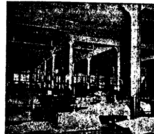
After Luxfer Prisms Installed.
