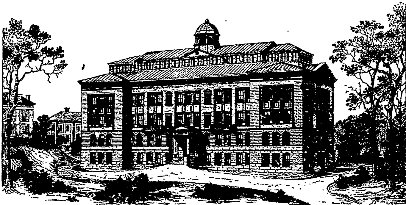
MCDONALD TECHNICAL BUILDING, MCGILL UNIVERSITY, MONTREAL.
