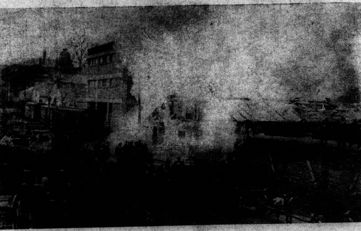
The above is the scene of last night's fire on Colborne street, when the Anguish livery barn was destroyed by fire. The building was one of the city's landmarks, and will be replaced by a modern structure.
