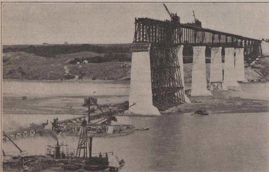
Completed C.P.R. Bridge Across the South Saskatchewan River.
