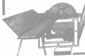
Bell's Feed Cutters are fitted with the La Marshe Knife. They cut cleaner, quicker, and hold their edge longer, than any other. They cut full mouth or a few straws equally well.
