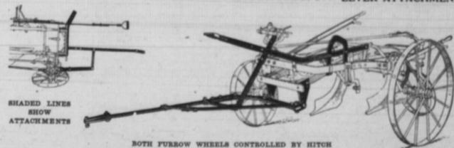
Adapted to any new Deere Gang. The John Deere Small Tractor Hitch and lifting lever attachments provide the farmer with an engine and horse plowing outfit in one implement.
