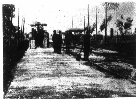
FIG. III.—PORTION OF ROAD ALMOST FINISHED.
