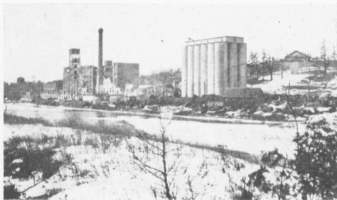
Fig. 2. View of the plant after the fire.
