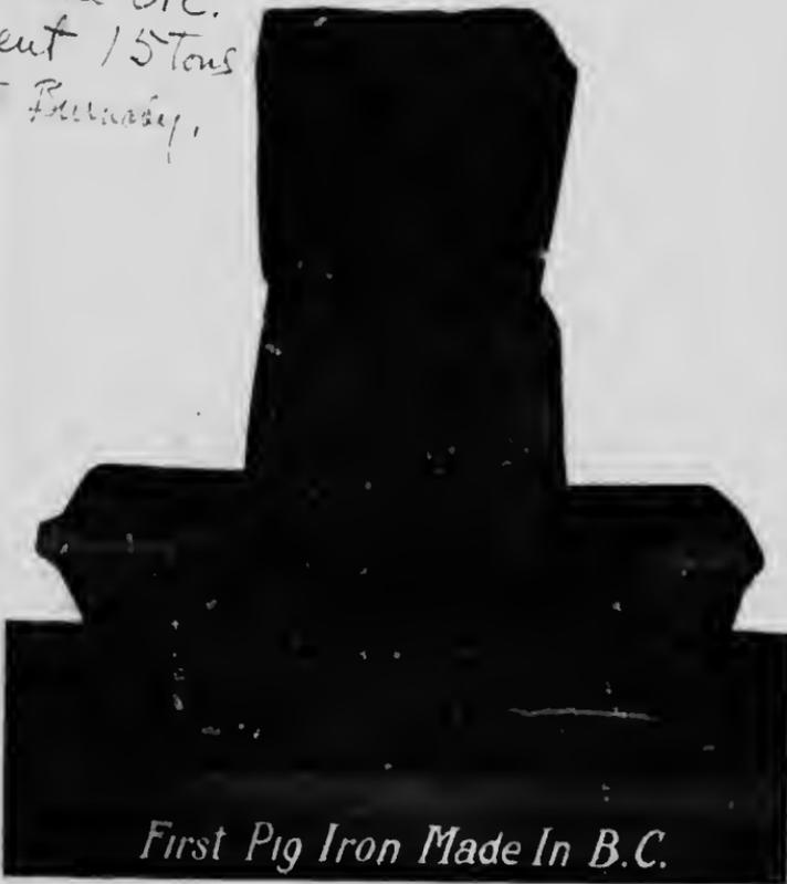
The above high-grade No. grey pig-iron, entirely free from all sulphur by analysis and produced solely from pure Texada Island, B.C., magnetite iron ores, was smelted by the above company in September, 1919, at the B. C. Electric Railway Company's Burnaby power house, being first fused in an electric furnace and then reduced by the duplex process.
