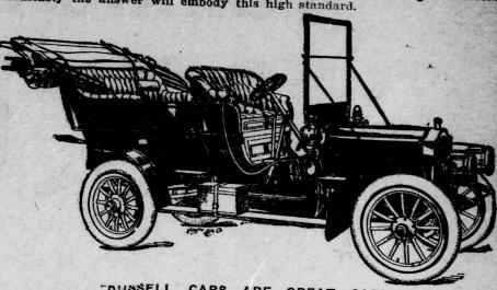
RUSSELL CARS ARE GREAT CARS." IN THREE MODELS. In each the metal to metal disc clutch, shaft drive, selective sliding gear transmission, nickel steel in all gears and shafts, powerful double brakes on rear wheels, positive lubricating and water cir-
