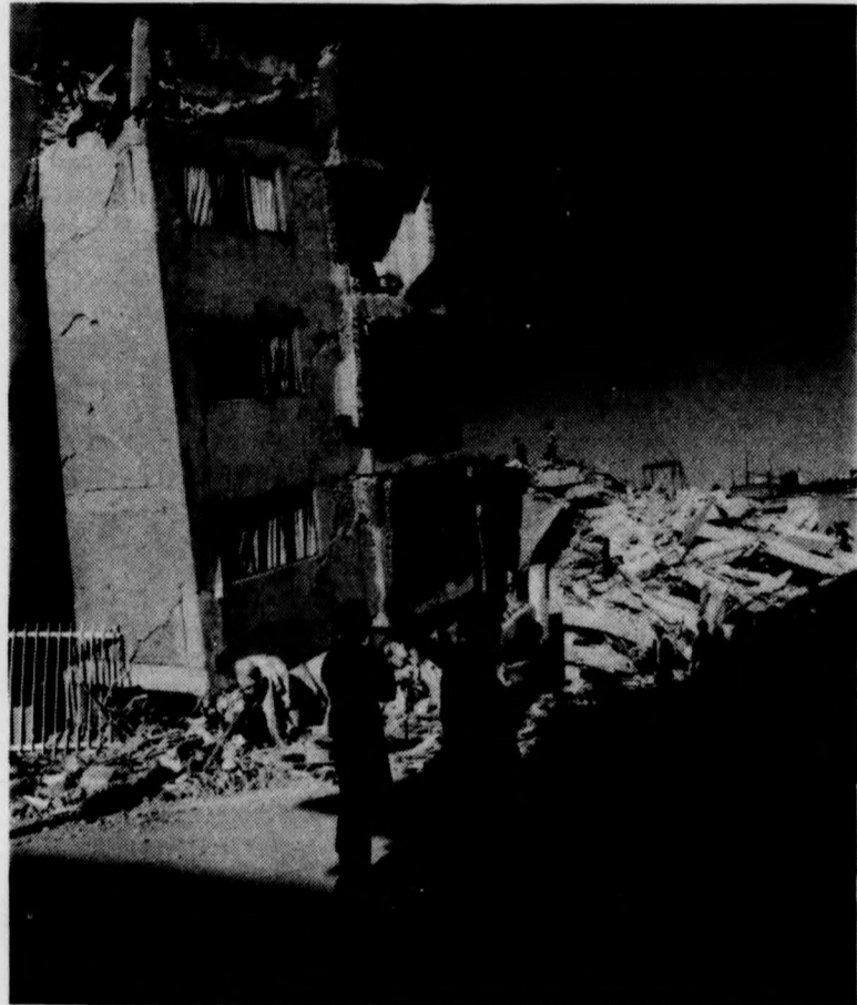
Housing which the government built was literally demolished by the earthquake, killing thousands of Mexicans due to the structures' poor construction.
