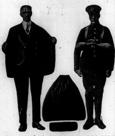
The new self-fitting inflated life-saving device, called the S.O.S. Emergency Life Belt; the invention of a Canadian engineer. The Belt under any and all conditions enables the wearer to remain upright with head well above the water surface. The views show Belt concealed under garmentinflated, ready for use in 20 seconds-converted to pillow and folded to pocket size; weight being 16 ounces-a particularly useful adjunct to the soldier's equipment.
