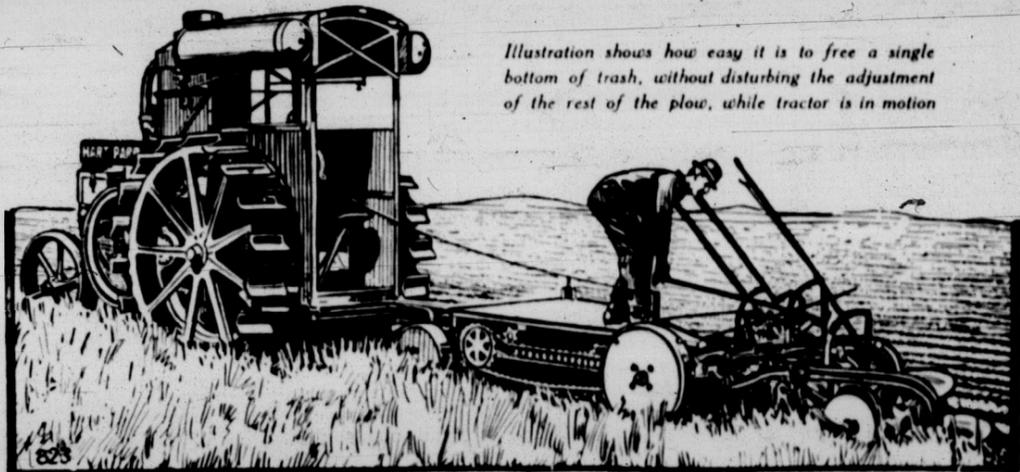
Illustration shows how easy it is to free a single bottom of trash, without disturbing the adjustment of the rest of the plow, while tractor is in motion
