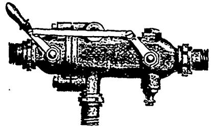
Will lift 25 feet and take water at 150 degrees. Only one handle to start and stop. No valves to regulate. Larger than any other Injector in the market. Prices and particulars on application to
