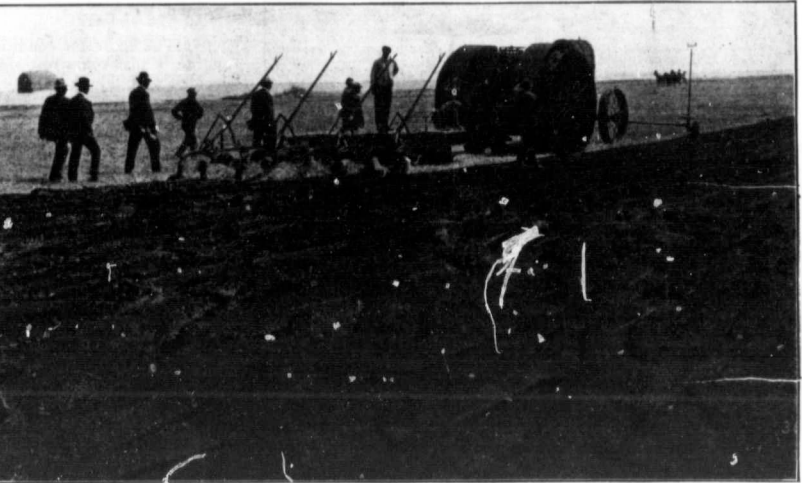
The Gas Tractor "Big 4 30" pulling 8 John Deere bottoms (Gold Medal Winner Class C).
