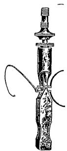
Our illustration shows a little tool of interest to opticians that has just been placed on the market by W. G. Fay, Springfield, Ohio. Its object is to facilitate lens setting, and it is said to be very effective for this purpose. It is easy of manipulation, and greatly assists in placing the lens in the frame and keeping the screw and temple from falling out. It is specially adapted to gold filled rid-
