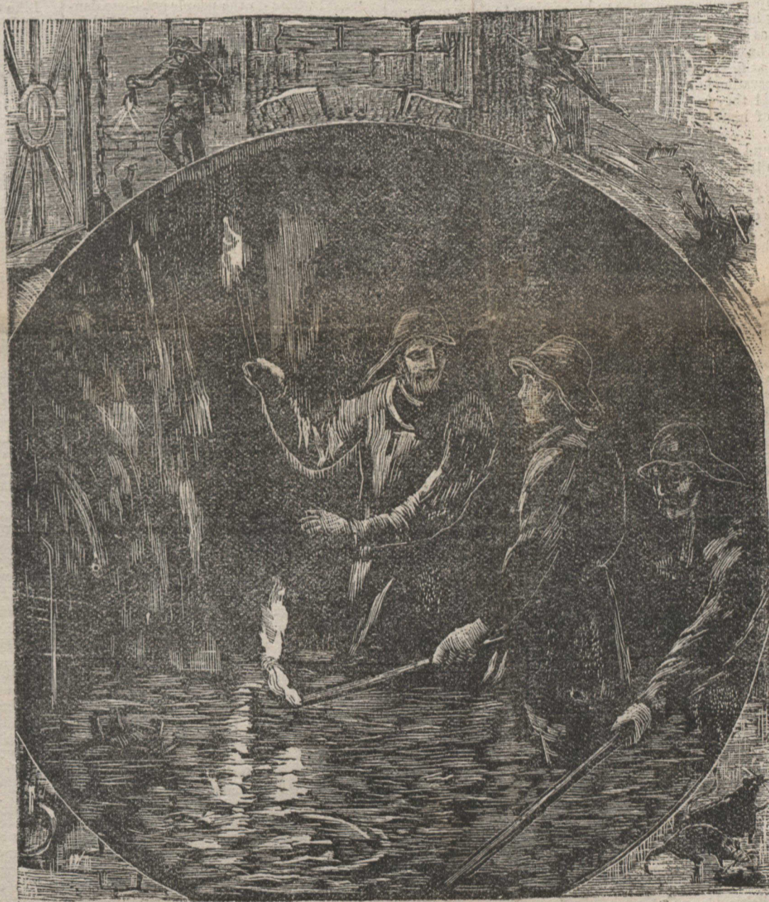
IN THE LONDON SEWERS.
