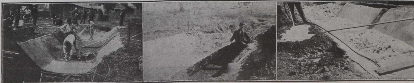
Filling Trench to Apply Hydraulic Head.
