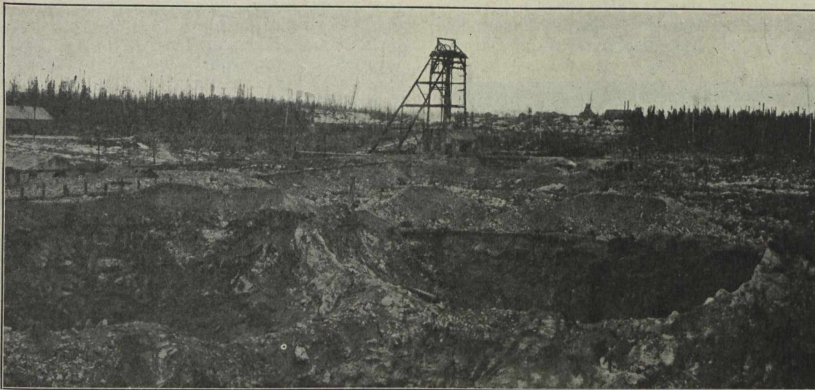
View Across Open Pits Towards No. 2 Shaft, Dome Mine.
