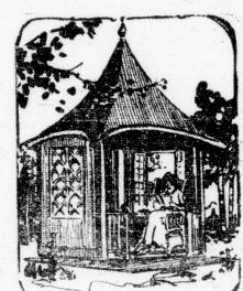
The newest things in summer houses and outdoor sleeping shelters are the revolving kind. These are made easily Design the sort of summer house you want, only don't attach it permanently to the foundations. Build a platform of good stout timber on the usual foundations. Fasten a steel rod at least an inch in diameter in the centre. The rod can be as long as desired. Get a dozen or more substantiallybuilt steel casters and attach them to the bottom of the summer house. In
