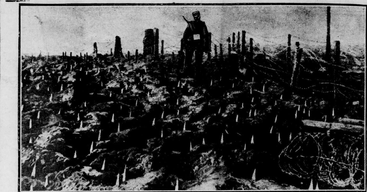
Staked Pits, with Wire Entanglements; a Deadly Device Used by the Austrians. This is a form of field-obstacle, turned to account on occasion in conjunction—as seen in the photograph above—with barbed-wire entanglements. The pits are of different depths and at irregular intervals, and where a number of men are available for the digging, can be excavated and staked in no long time. The obstacle is ordinarily laid down as close range of the defenders' firing-line as possible, to impede any attempt to "rush" the position and hold the assailants back, checked and "hung up," as it were, all the time under fire, so that the bullets of the defence may do their deadly work. In the fighting in the Austrian Danube provinces and on the Serbian border, obstacles such as these have been largely employed.
