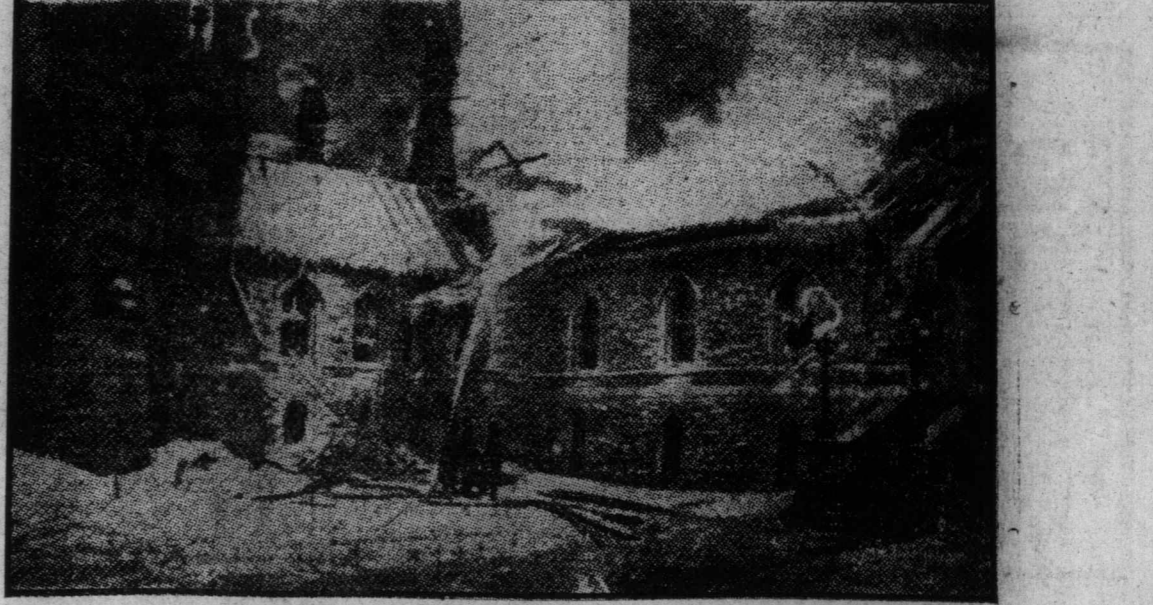
Firemen playing hose on the wing leading to the Library which was eventually saved.
