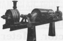
Two Worthington 3-Stage Turbine and McCormack Water Wheels, built for Port Arthur, Ont., Water Works, 1440 gal. per minute against 350 ft. head.
