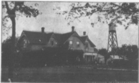
In this house there is water on tap. The windmill on the barn is geared to elevate water to the raised tank. Note that the well is protected by the pump house.
