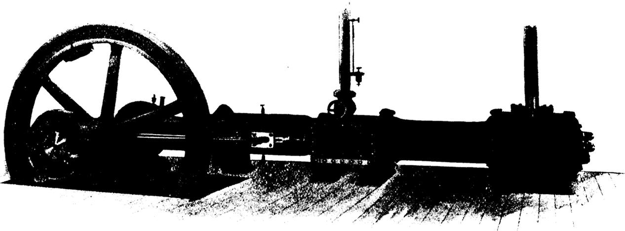
This cut illustrates the first half of a Rand class "B" air compressor. We recommend the installation of a first half whenever there is a probability of increased capacity being required later on. When second half is added, machine can be compounded on the steam end, on the air end, or made compound steam and compound air.
