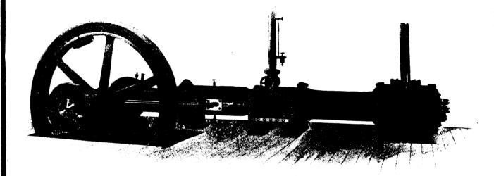
This cut illustrates the first half of a Rand class "B" air compressor. We recommend the installation of a first half whenever there is a probability of increased capacity being required later on. When second half is added, machine can be compounded on the steam end, on the air end, or made compound steam and compound air.
