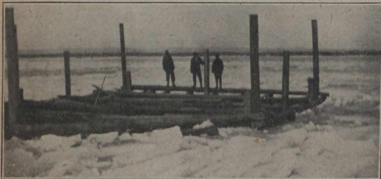
Nose of Protection Pier ready to sink.
