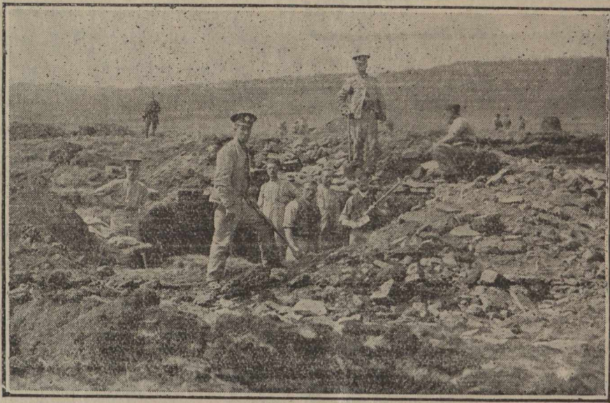
Engineers Trench Digging at Buxton.
