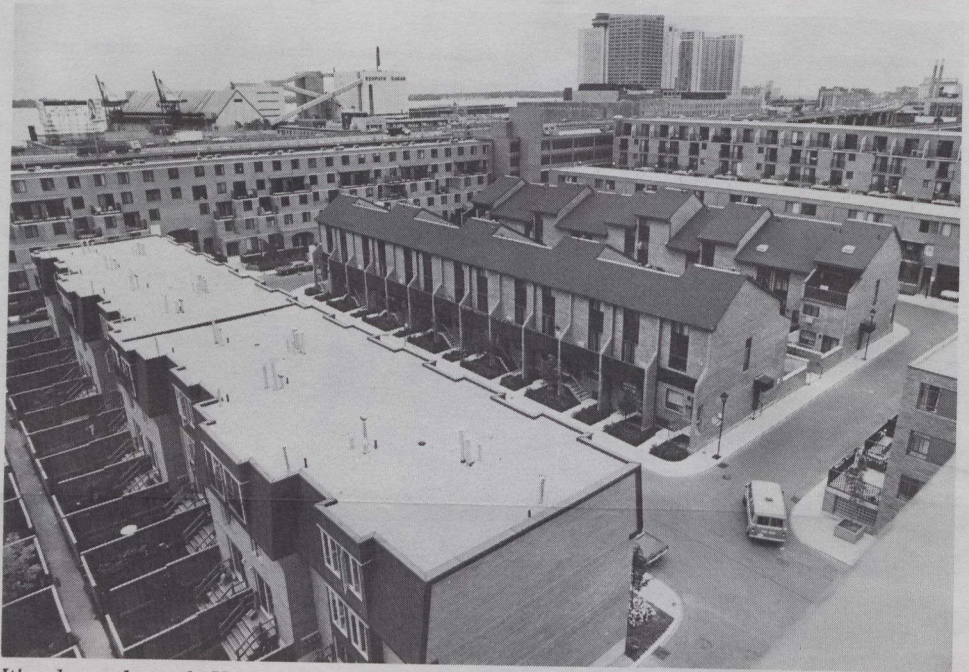
Woodsworth and Harmony Co-operative townhouses, with Cathedral Court Homes apartment, Gardiner expressway and Toronto harbourfront (upper left).
