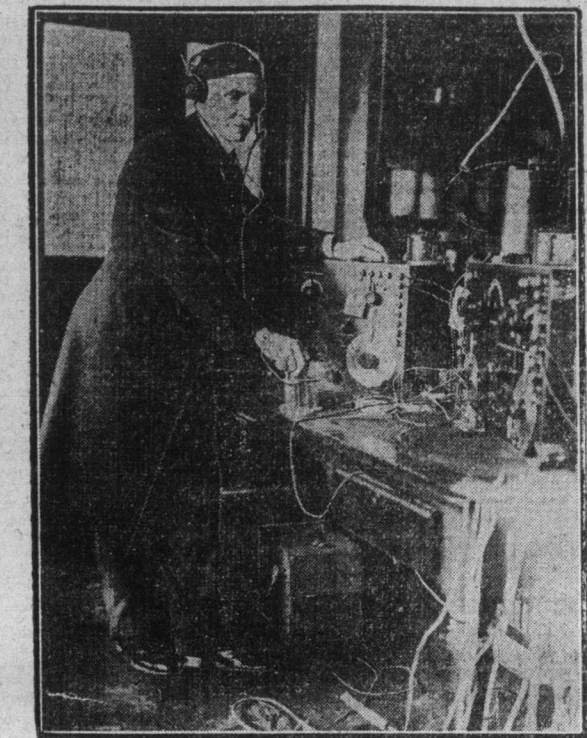
INVENTOR OF UNDERGROUND RADIO SYSTEM. James Harris, Rogers, of Hyattsville, Md., is the inventor of an underground radio system, by which wireless messages may be sent and received underground or water without the use of aerials.
