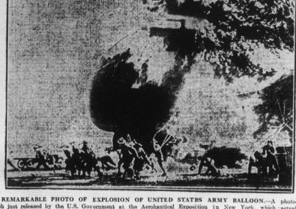
graph just released by the U.S. Government at the Aerohautical Exposition in New York, which actuall shows what happened when a kite balloon, inflated with hydrogen gas was ignited by the static cause by a soldier's hair brushing against the bag. A special non-inflammable "Helium" gas now being tried, elim inates the possibility of such an occurrence as above.
