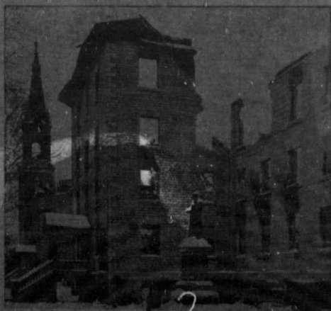
View of part of the Main Building in ruins.
