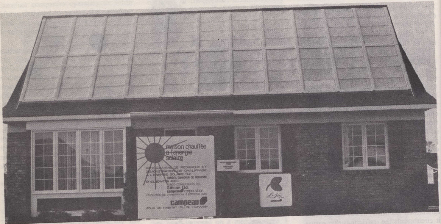
This Campeau Corporation design at the Ile Brizzard development in Laval, Quebec features an air-rock solar energy system.
