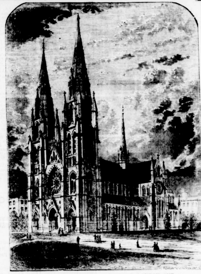
THE NEW ST. PETER'S CATHEDRAL, LONDON, ONT.
