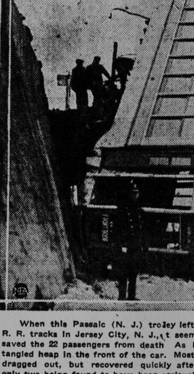
When this Pascale (N. J.) trolley left the trestle over the West Shore R. R. tracks in Jersey City, N. J., it seemed that a miracle was all that saved the 22 passengers from death. As it was, all were hurled in a tangled heap in the front of the car. Most of them were unconscious when dragged out, but recovered quickly after being taken to the hospital, only two being found to have been seriously injured.
