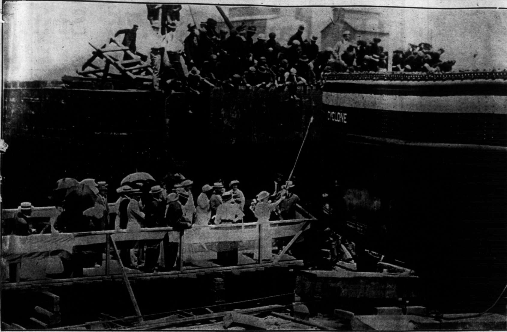
THE LAUNCH OF THE WORLD'S LARGEST DREDGE. A SCENE IN THE POLSON SHIPYARDS, WHEN "CYCLONE," WHICH WILL BE USED ON TORONTO HARBOR IMPROVEMENTS, STARTED TO SLIDE INTO THE WATER.
