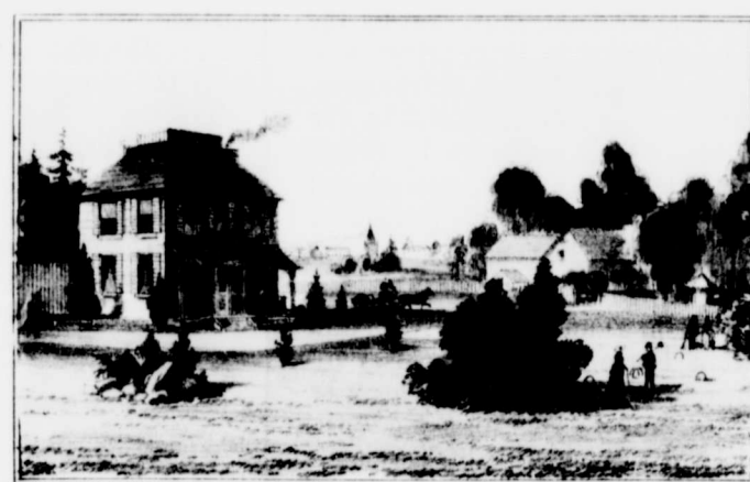
IMPROVED HOUSE FINISHED
