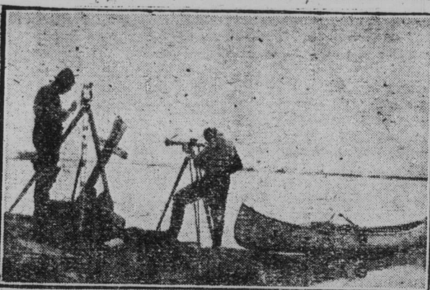
Surveyors of the Topographical Survey of Canada at work in northern waterways of Manitoba. The instrument to the left is a transit-theodolite, and that to the right is a ranger-finder.
