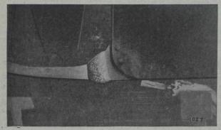
Sternshoe of a Vessel Welded With Thermit, and the Vessel Was Taken Off the Drydock in Less Than Three Days.
