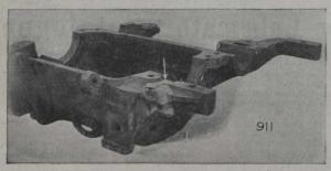
Motor Cases Can Be Welded With Thermit in a Few Hours, and Kept Them From the Scrap Heap.
