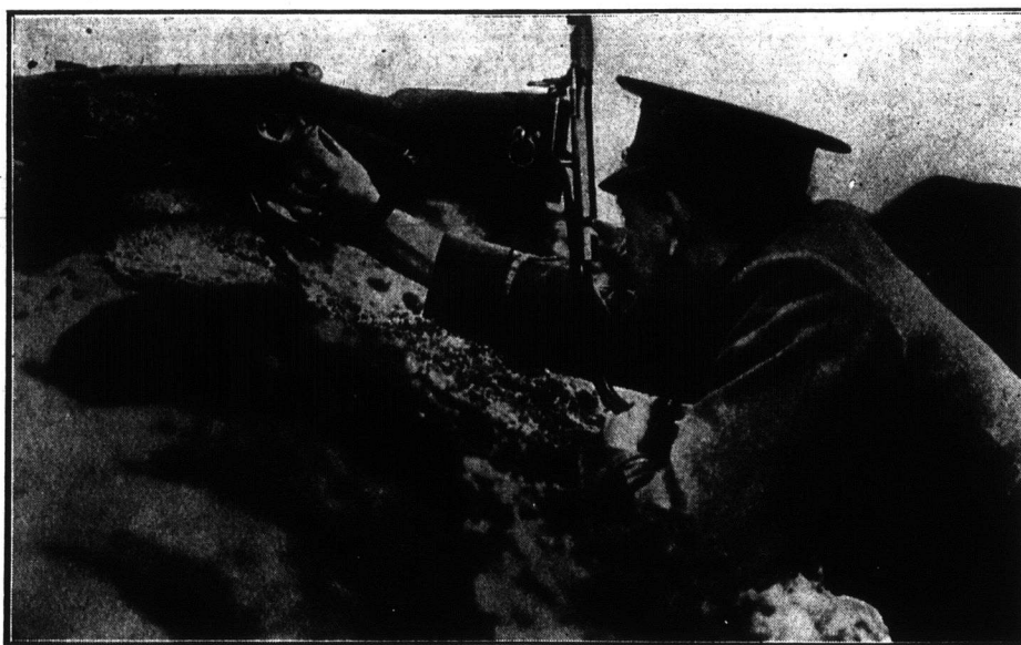
Dutch soldier firing rifle, using the "Erasmus" periscope. This device was designed by J. H. Erasmus, a Dutch inventor, and is named in his honor. It is attached to the butt of the rifle and enables the soldier in the trench to aim and fire accurately without danger of death from the enemy's bullets. It is in use in the Dutch army and should revolutionize sniping along the battlefronts.
