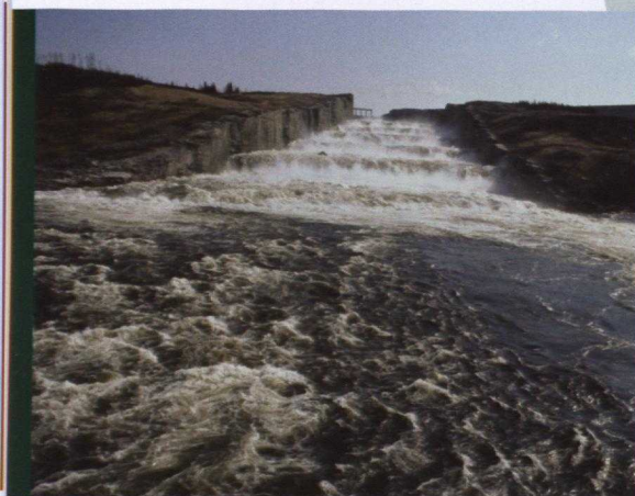
The Robert Bourassa dam. Hydro-Québec's La Grande complex is the world's largest hydroelectric generating system.
