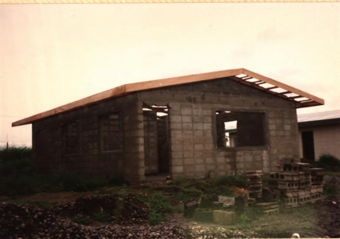
No. 66. Door and window framing underway.
