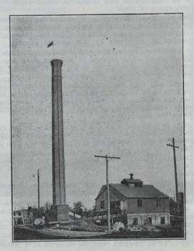
This Ideal High Temperature Destructor during the Demonstration Test consumed 15 tons of garbage in 8 hours, and one horse weight, 1385 lbs., in 20 minutes.
