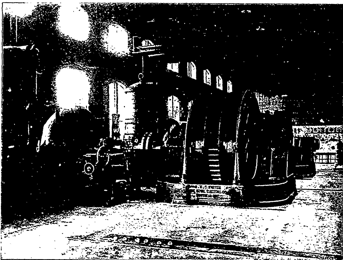
1000 K.W. "S.K.C." DIRECT CONNECTED UNITS—CATARACT POWER COMPANY'S PLANT.
