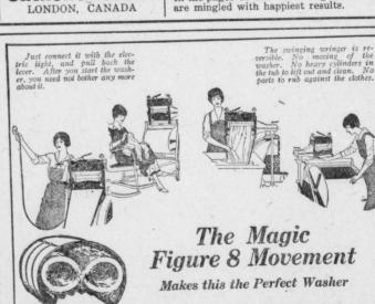
All washing machines cleanse the clothes by forcing the water back and forth through the material. But in the 1900 Cataract Washer the water swirls through them in a figure 8 movement which forces it through them four times as often as in the ordinary washer!
